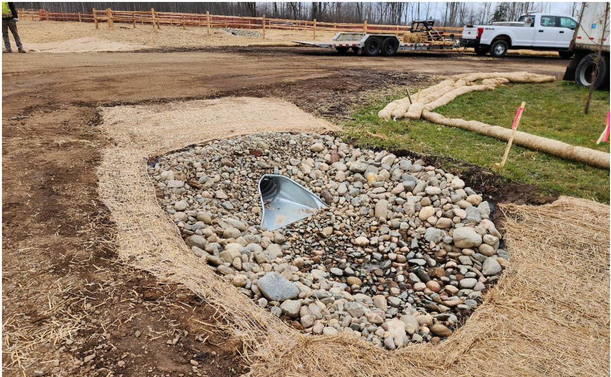
Photo 5: Campground Stormwater Treatment Pond and Culvert at Prior Trailhead Area
