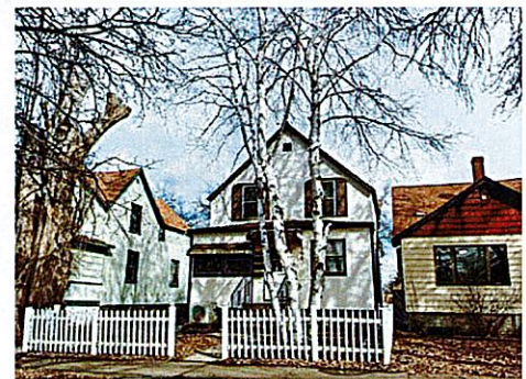
Existing single family homes
