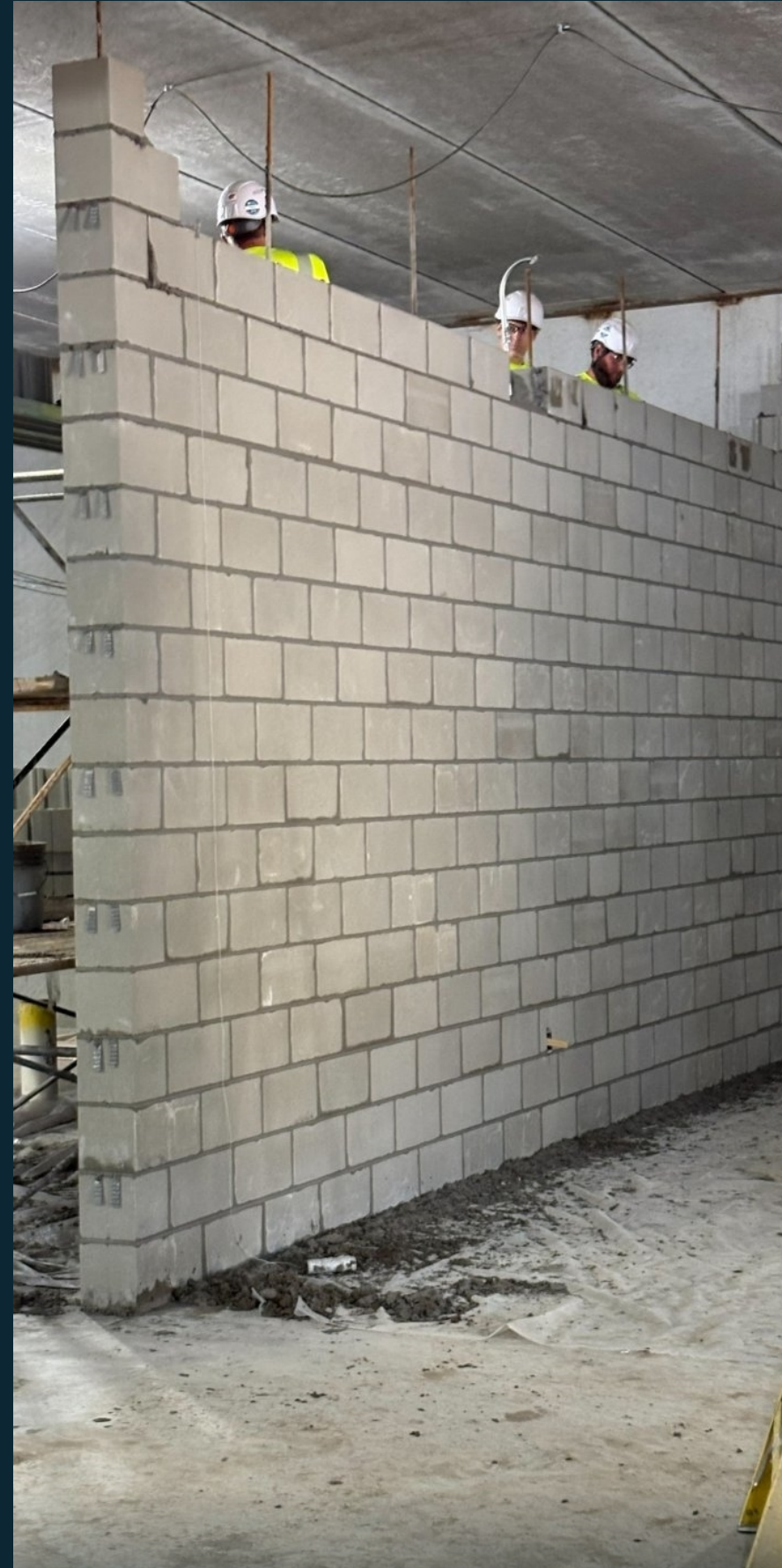
CMU partition walls being laid on the
