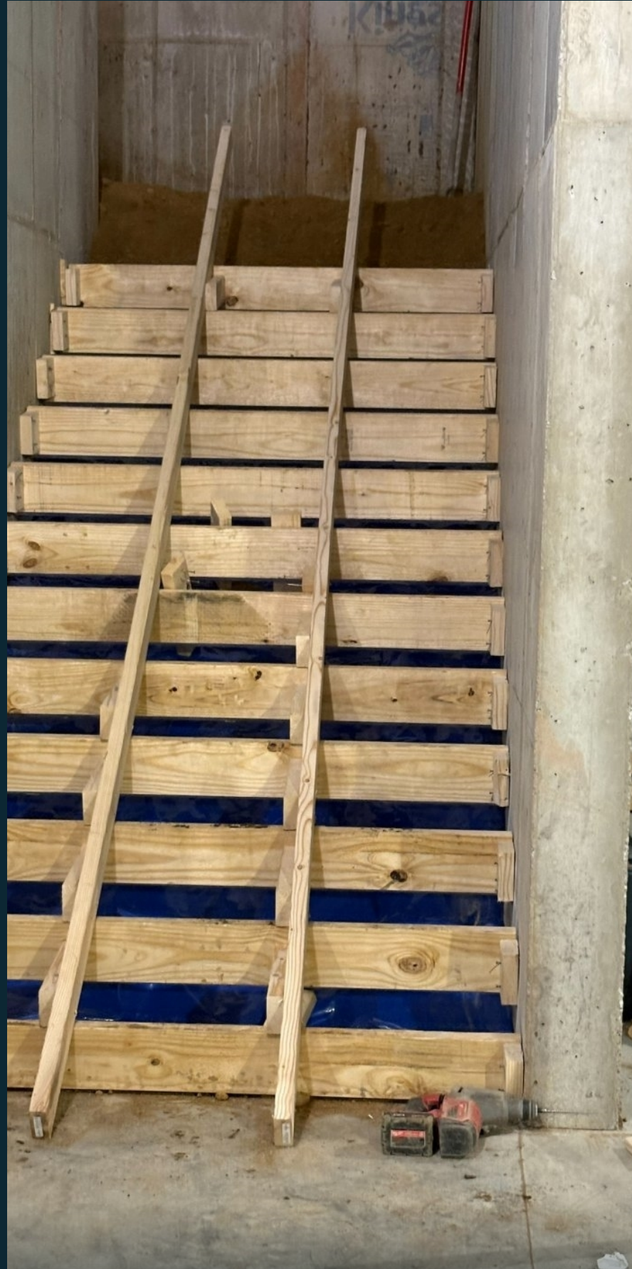
Cast-in-place stair forming at the
